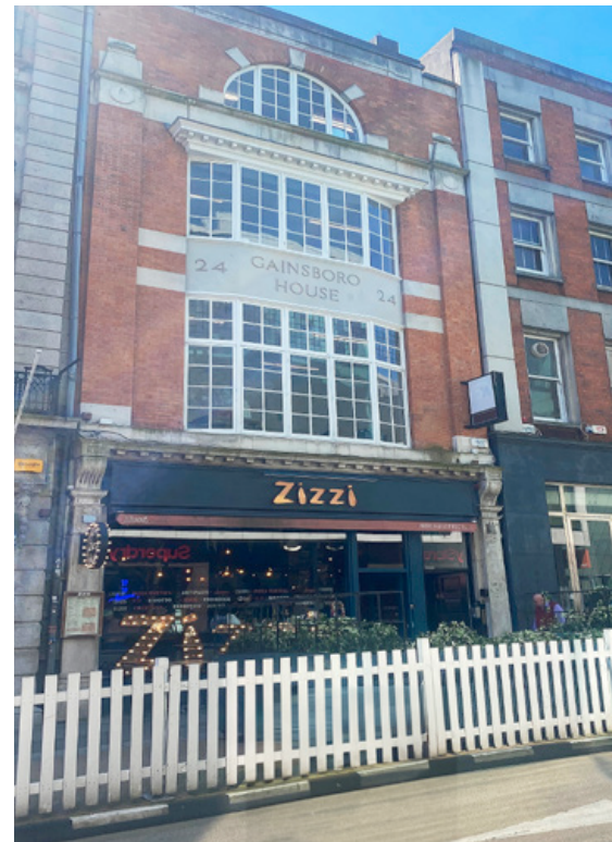
ABOVE: 24 Suffolk Street, Dublin 2
